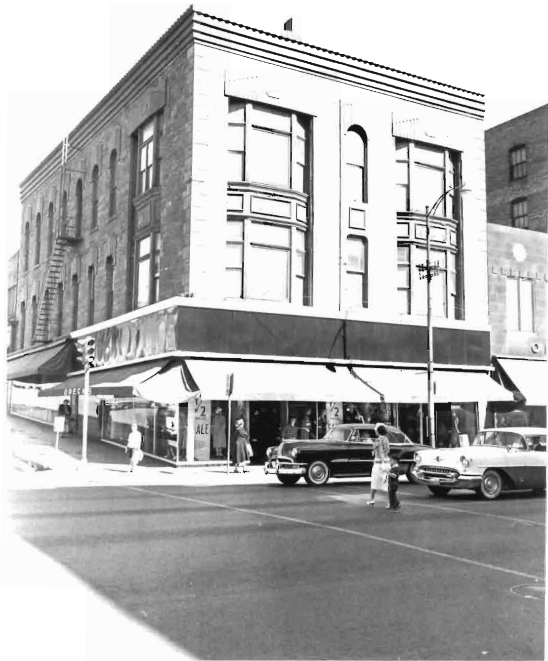
Oreck's Department Store as it appeared in 1958. Founded in 1909 by Gabriel and Lena Polinsky Oreckovsky, this was originally the "Hunter Block," architecturally modified several times by the Oreckovskys. (Source: Northeast Minnesota Historical Center)
