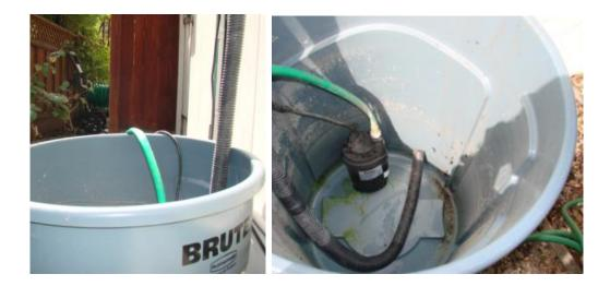
B. Attach the sump pump to the hose reel cart with a short length of hose.
